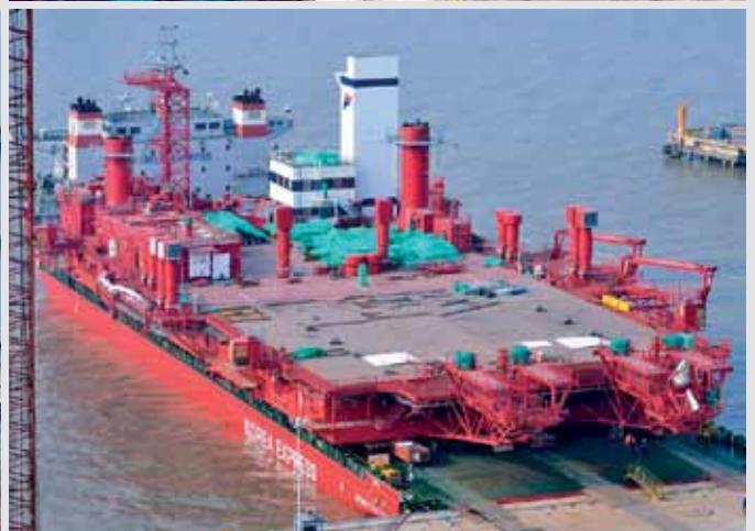
Roll-on operation for the 5,400-tonne upper hull block to be loaded onto the barge for delivery to Keppel FELS
