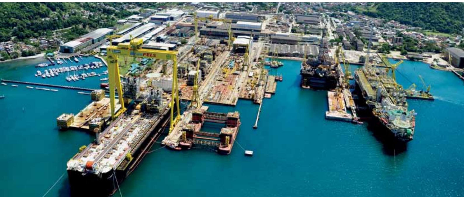
BrasFELS completed the first lifting campaigns for two Floating Production Storage and Offloading (FPSO) vessels in January
