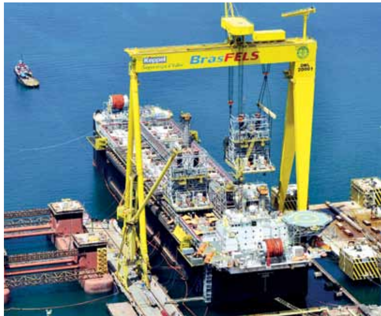
BrasFELS' 2,000mt gantry crane was utilised to carry out the first lifting campaign for P-66
